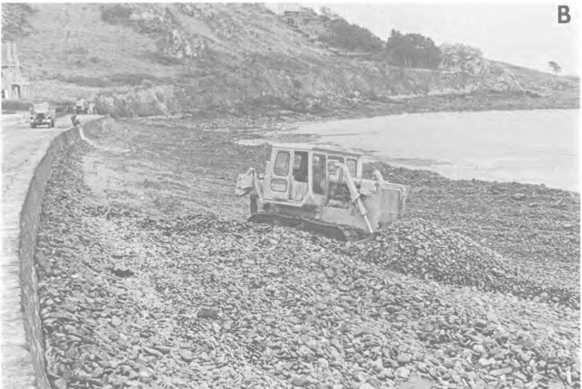
Figure 4-55. (A) Heavily oiled cobbles of station AMC-16 were pushed into furrows to aid cleaning by wave action. (B) At station F-80, a similar method of clean-up was in operation.
