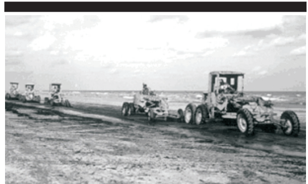
Figure 2. Use of road graders on hard-surface, fine-grained sand beach at the Alvenus spill, Texas.
