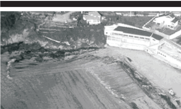
Figure 5. Early use of berm relocation in 1976 to naturally cleanse oiled sediments at the Urquiola oil spill.
