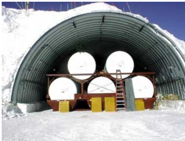
Figure 8. Photograph of the end view of the fuel storage pods during construction.
