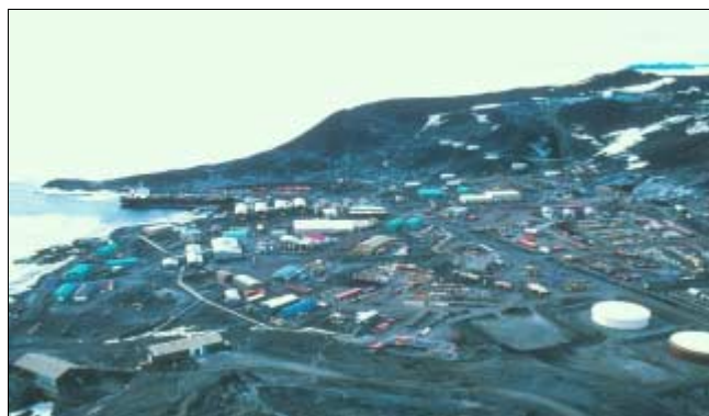
Figure 3. McMurdo Station, Antarctica. The old tank farm in the upper right is being replaced with new bermed tanks in the lower right. The sole tanker calling each year at McMurdo is offloading, left center of the photograph.
